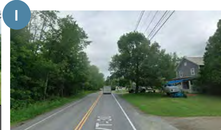
I Shift pavement and centerline 7 ft to avoid stone walls and houses on east side while minimizing impacts to west side.
