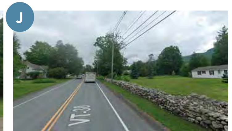
J Remove or relocate ~70 ft of stone wall at 1148 VT-30 (Misai & Misai) currently located within 2 ft of pavement edge
