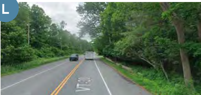
Existing pavement widens from here to the south. Shift lines on existing pavement to re-allocate extra space for pathway on east side. Widen as necessary. Trees will be impacted, particularly outside of 612 VT-30.
