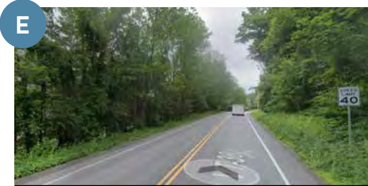
Existing road is not centered within right-of-way due to slopes on the west side. Build path to right-of-way edge without barrier but no grass buffer.
