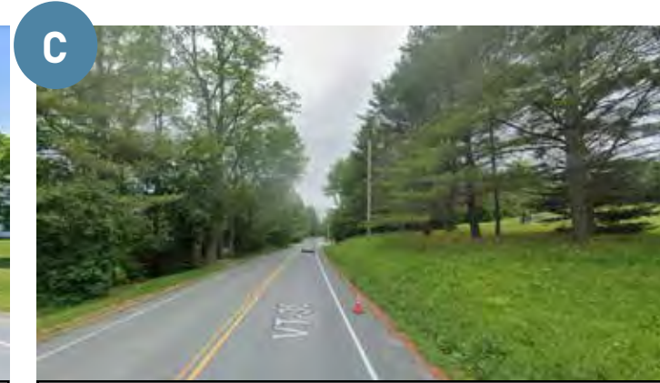
Shift pavement and centerline 5 ft to avoid steep slope and trees on east side. OR: if property owner is supportive, acquire easement, remove 11 trees and re-grade slope.
