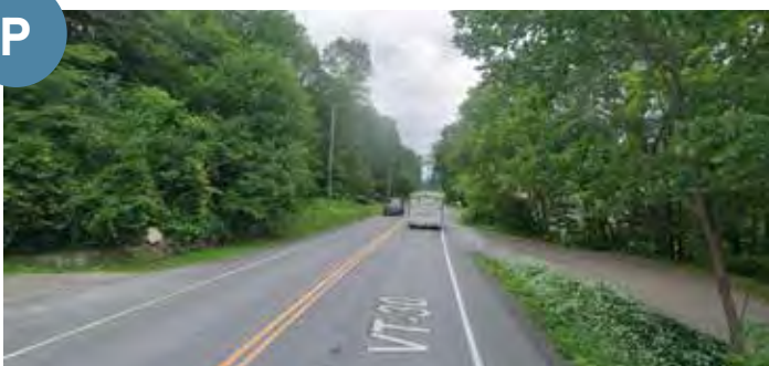
Shift centerline by 3 ft to reduce slope impacts on east side while avoiding stone wall on west side. Re-grading of driveway and retaining wall may be needed.
